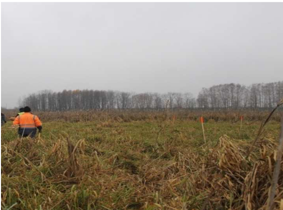
Figures 17 and 18. The boundaries of the planned water bodies are marked in the field with painted stakes (Photo: U. Valainis)
