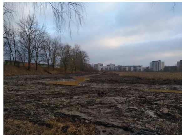
Figures 19 and 20. Excavation and levelling of aquatic vegetation, silt and soil material performed in accordance with boundaries put in nature (Photo: U. Valainis)
