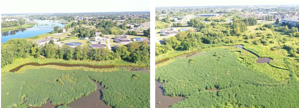
Figures 25 and 26. Bird's eye view of the pond/canal system created in the Esplanade Wetland (Photo: M. Nitcis)
