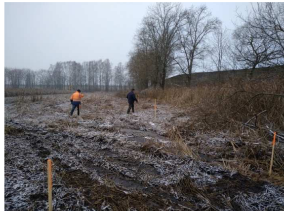
Figures 17 and 18. The boundaries of the planned water bodies are marked in the field with painted stakes (Photo: U. Valainis)
