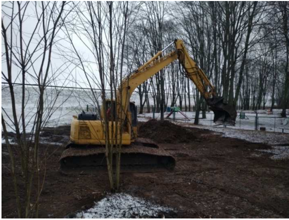
Figures 6 and 7. Where tree stumps could make future management difficult, tree stumps and roots are removed (Photo: U. Valainis)
