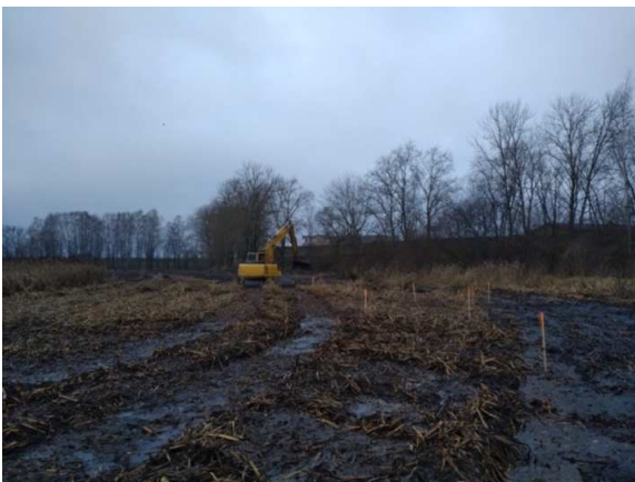
Figures 19 and 20. Excavation and levelling of aquatic vegetation, silt and soil material performed in accordance with boundaries put in nature (Photo: U. Valainis)
